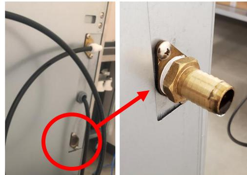
2. The provided drain kit consists of the Molded Drain Line, 3 worm gear clamps, and one female  $\frac{3}{4}$ " NPS x 1" Barb fitting that will accept  $\frac{3}{4}$ " NPS x  $\frac{1}{2}$ " CTS.
